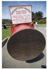
The weight of the roadway is hung from two cables that pass through the two main towers and are fixed in concrete at each end. Each cable is made of 27,572 strands of wire. There are 80,000 miles (130,000 km) of wire in the main cables.
